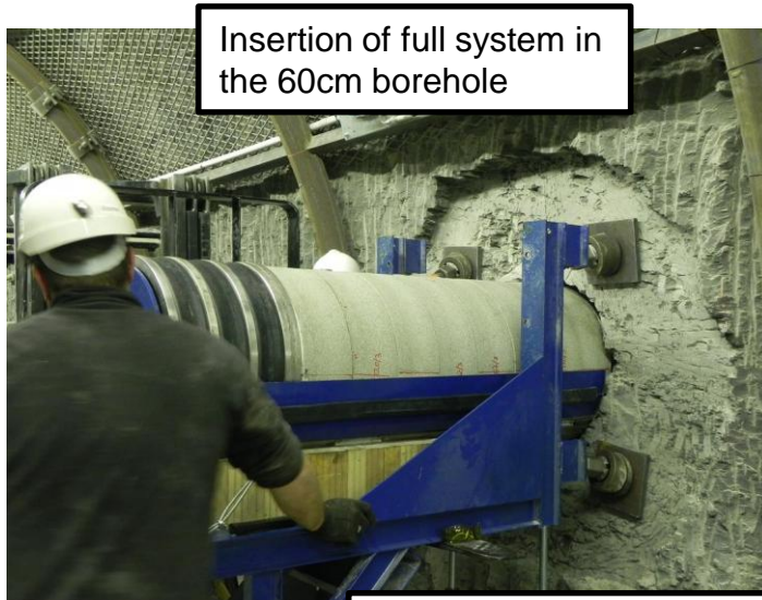
Central tube with all cables and lines running, and with the 4 anchors
