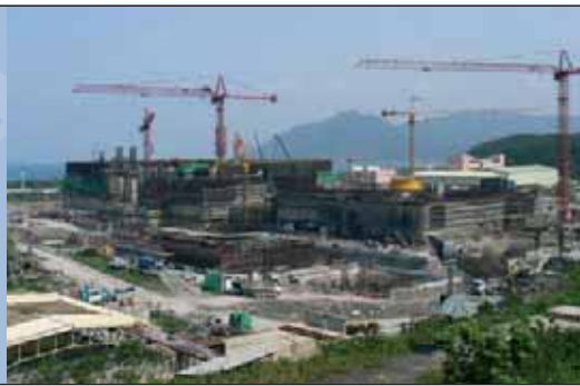
Lungmen Nuclear Power Plant
