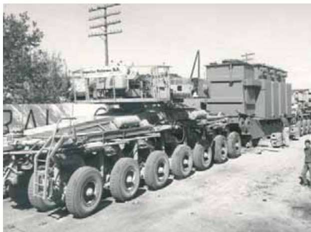
Transport used during the construction of José Cabrera Nuclear Power Plant
