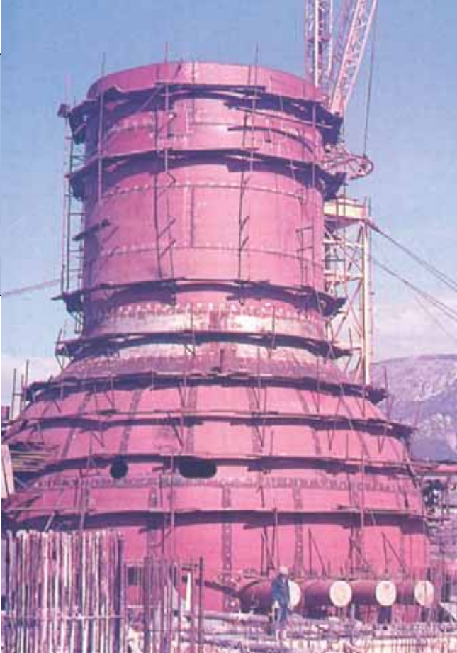
Construction of Santa María de Garoña Nuclear Power Plant
