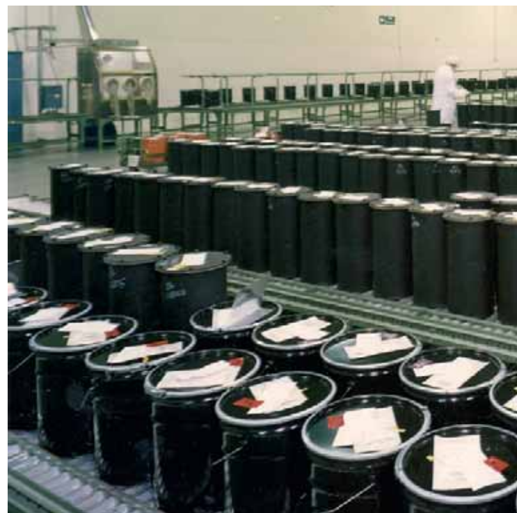
Fuel elements production facility in Juzbado
