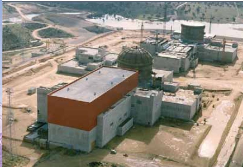
Construction of Valdecaballeros I and II Nuclear Power Plant
