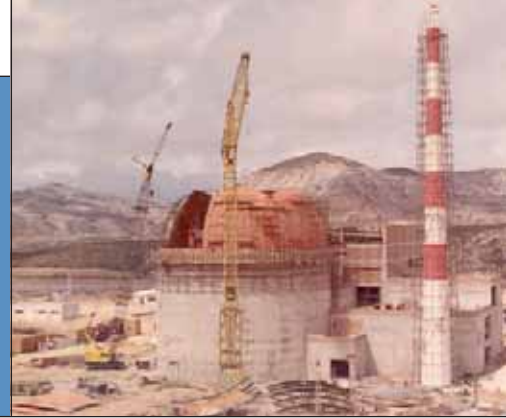
Construction of José Cabrera Nuclear Power Plant
