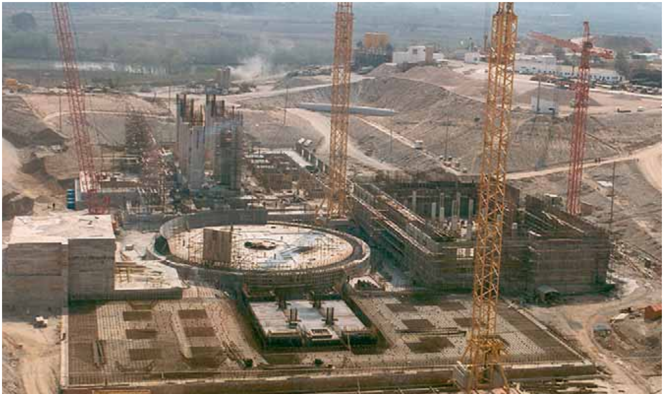
Construction of Ascó I and II Nuclear Power Plant
