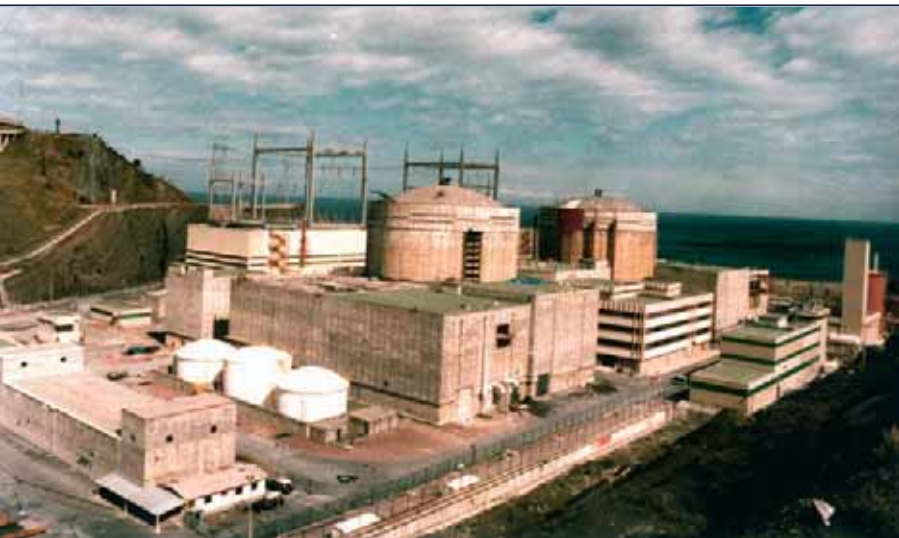
Construction of Lemóniz I and II Nuclear Power Plant
