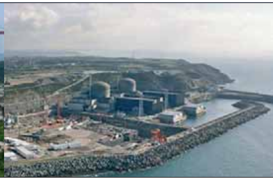
Flamanville Nuclear Power Plant
